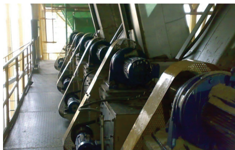
Bagasse Feeder Conveyor
