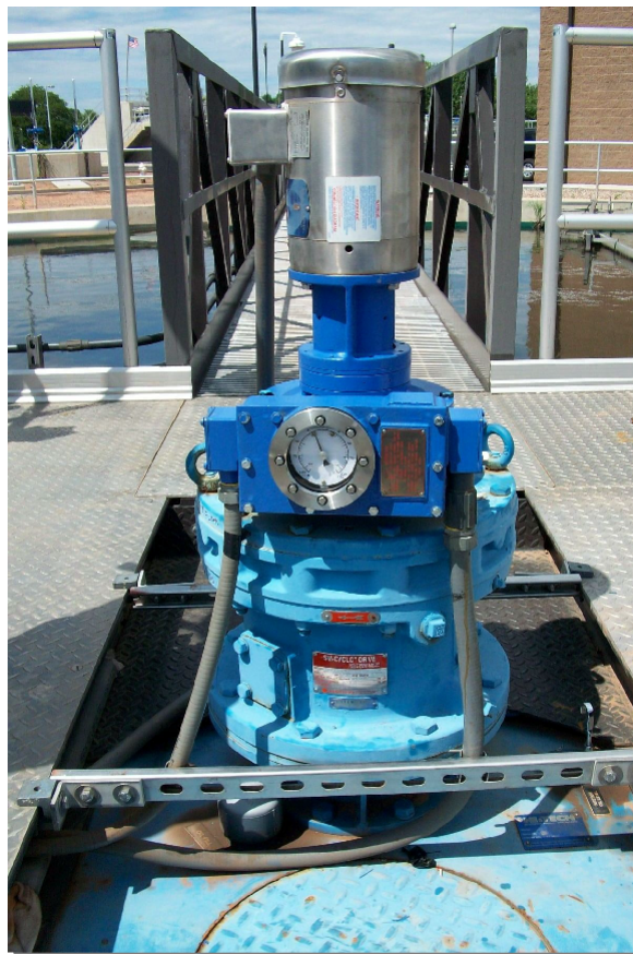
Figure 8. This Cyclo ® speed reducer by Sumitomo Drive Technologies is equipped from the factory with an optional torque limiter wired into the systems control circuitry to shut the system down when overload occurs. The analog gauge provides jobsite personnel with a quick and easy access view of the loading conditions while the unit is in operation.
