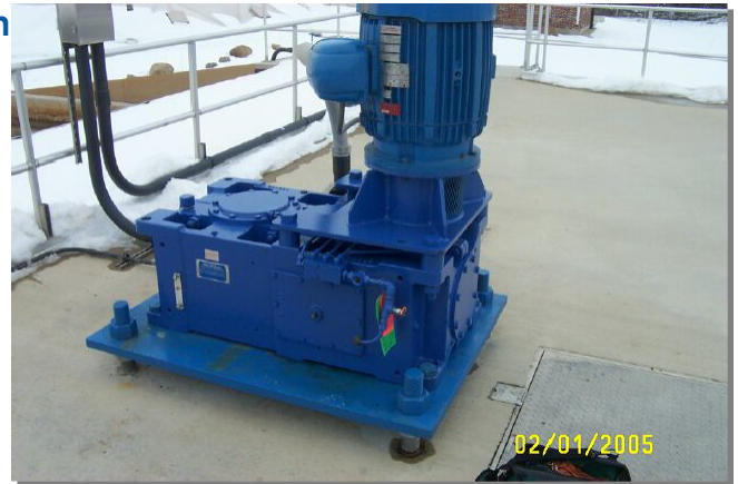
Figure 5. Parallel reducer installed above an impeller shaft with a flange-mounted motor connected to the top of the reducer via a motor lantern.
