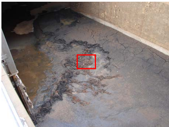
Figure 6. Aerator 1 Basin Sediment
