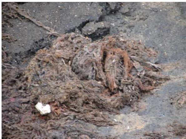
Figure 7. Detail of Fibrous Debris in Aerator 1 Basin
