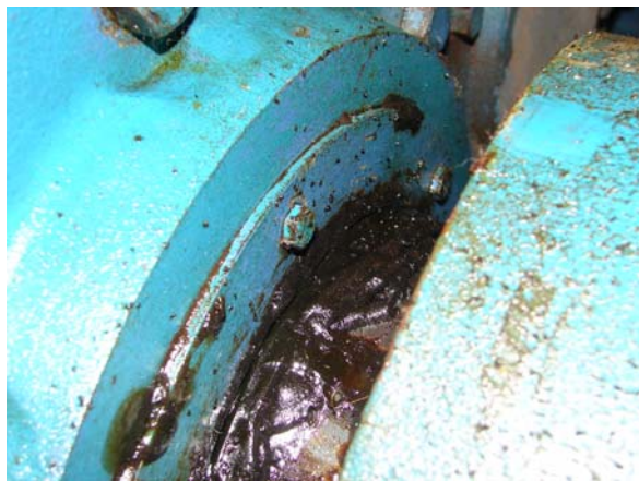
Figure 10. Low Speed Seal Area at Factory Inspection
