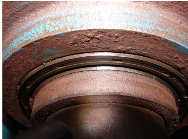
Figure 11. Input Shaft Seal Area at Initial Inspection
