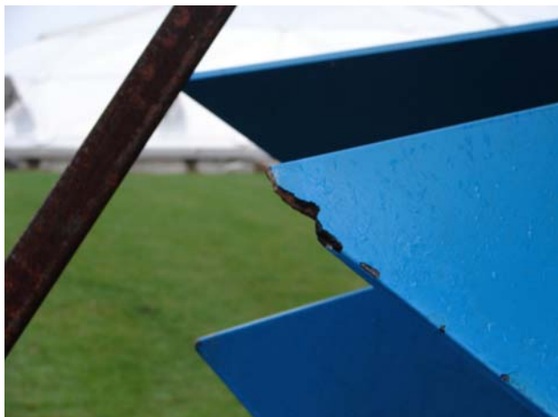
Figure 8. Example of Broken Impeller tip for Aerator 1
